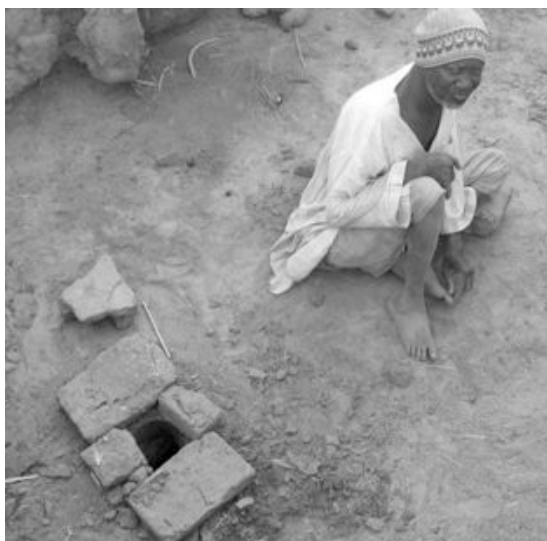
Figure 6.6 This disabled man, with limited use of his legs, must crawl on all fours to visit his traditional household latrine. Here he demonstrates how he temporarily places dried mud bricks around the latrine hole to better place himself for latrine use without becoming soiled.
