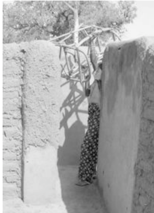
Figure 6.33 Wooden chairs must be built with the size of the latrine entranceway in mind; or latrine entrance ways need to be constructed to accommodate passage by assistive devices. This latrine chair must be lifted above the latrine entranceway.
