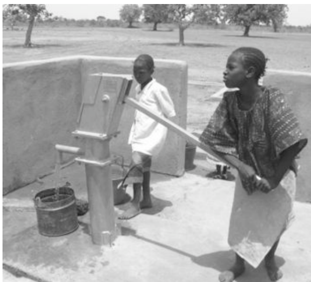
Figure 1.4 A typical hand-pump and superstructure facility of the Mali Rural Water Project
