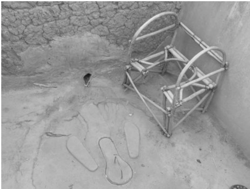
Figure 6.30 Wooden latrine chairs made with wire binding can be stored in the latrine area for easy access and use.
