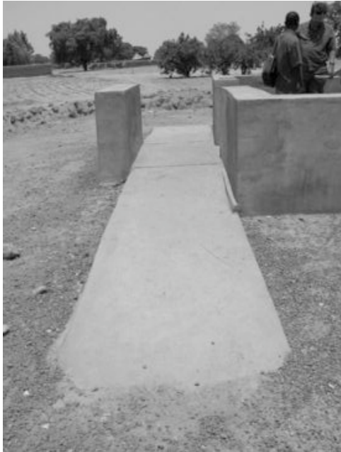
Figure 4.6 Pedestrian and tricycle access and egress ramp for a pump superstructure. Note the two parallel depressions at the top of the ramps for stabilizing the rear and forward wheels of a parked tricycle.
