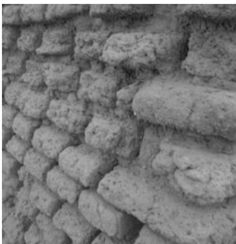
Figure 6.8 Exposed clay brick walls in the interior of latrines, while subject to deterioration by seasonal rains, can provide helpful handholds and support for some disabled and elderly persons.
