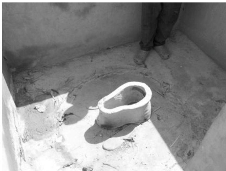
Figure 6.16 Terra cotta latrine seat in use on a sanplat latrine in the home of a polio victim. When not in use, the seat is moved to the side of the enclosure for storage.
