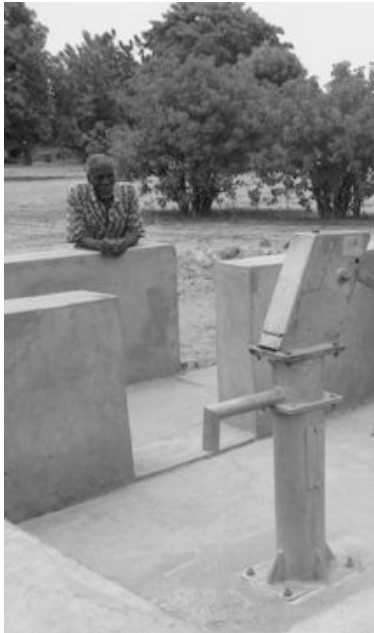
Figure 4.9 A pump superstructure apron filled to the same level as the pump support platform and the entrance ramp. Pump superstructures with no steps or abrupt elevation changes at the ground level can greatly enhance pump access by disabled persons. (Note: the shallow drainage channel running across the floor of the entranceway does not represent any change in floor level.)
