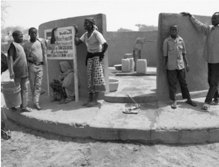
Figure 4.1 A hand-pump and protective superstructure in Niger, with two entry steps and a pump support platform inside the enclosure. A disabled member of the community can find the three steps challenging to negotiate, especially when carrying a container full of water.
