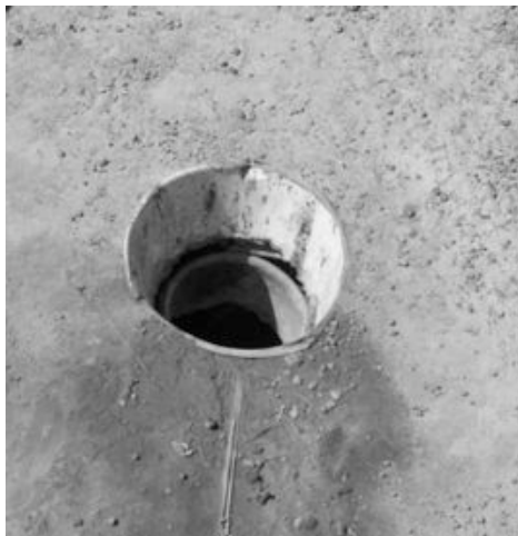
Figure 6.5 A traditional latrine used by a disabled person who, due to lack of adequate leg strength, must sit directly on the hole. Note the rim of the hole (the remains of an old metal container) is flush with the ground surface so as to minimize discomfort when the user is seated on the ground.
