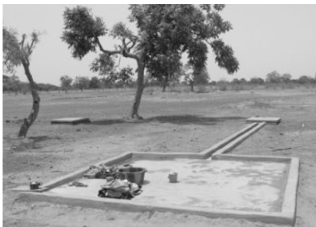
Figure 1.5 A typical laundry apron, usually placed within a few meters of the pump, which provides a convenient and hygienic place for clothes washing.
