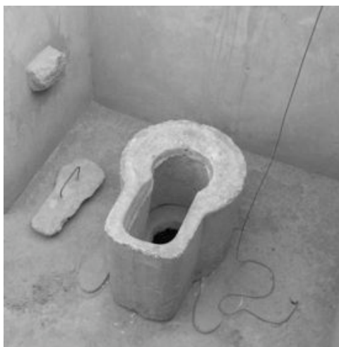
Figure 6.36 A cement latrine seat designed by WaterAid Mali for use by the visually impaired.
