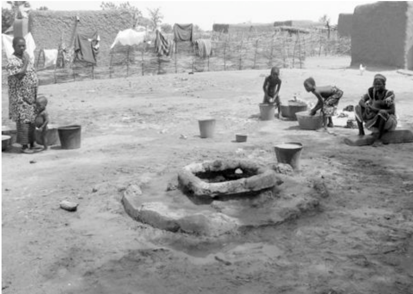
Figure 2.6 Traditional village well in south-central Mali. Note the poorly constructed apron and the standing water and mud surrounding the well.
