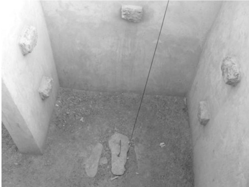
Figure 6.13 A sanplat latrine with cover, equipped with a vertically placed string for assisting the visually impaired in hole location and body positioning when squatting.
