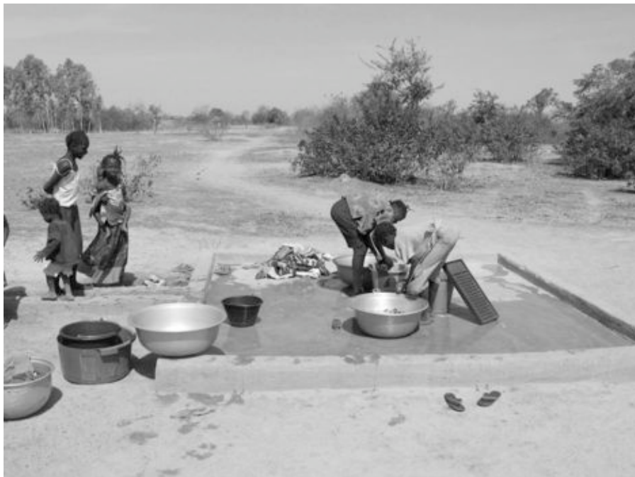
Figure 4.5 A well-used laundry apron in Mali. Many disabled persons are unable to stand and wash their clothes and must sit on the ground or on available seating. This apron provides no functional seating above the wet floor.
