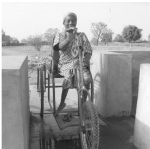
Figure 4.8 A disabled woman uses the access ramp to access the pump superstructure entrance.
