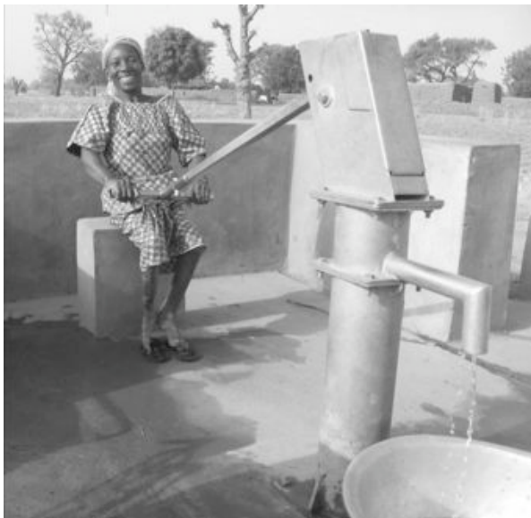
Figure 4.17 A woman with lower-body disability uses the completed combination of the end-seat and T-handle attachment.
