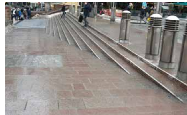
Outside Oslo central station, the edges of the steps were marked due to complaints of a breach of § 9 (© Berit Vegheim)
