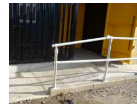
The City Bridge Trust funds access improvements for community organisations; for example, ramps and automatic doors for Archway youth club.
