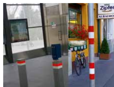
Indicating one of the best practices that were identified during the research process: clearly marking all potential hazards in the street to make them as visible as possible for persons with visual impairments.
