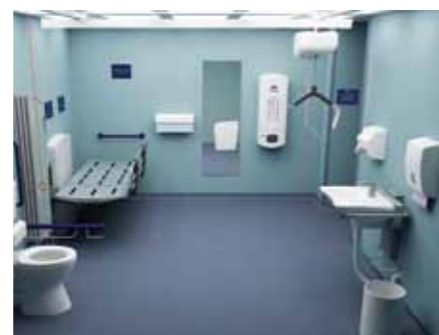
Changing Places toilets are different to standard disabled toilets – they include special equipment and are spacious.
