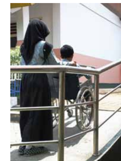
An external ramp linking separate school buildings. Madrassah Balarajam (Public Junior Secondary School), in Tangerang, Banten, Indonesia (© Maria Siahaan, AusAID)
